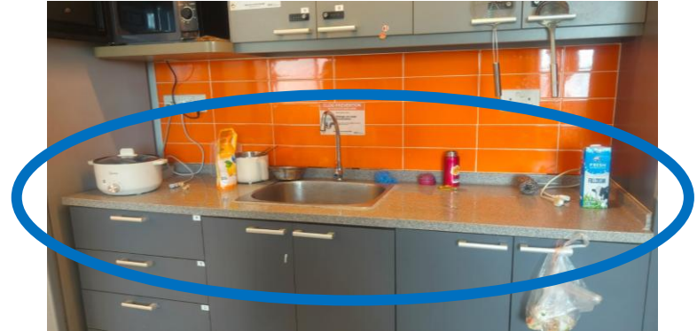
Wet Kitchen Countertop that caused short circuit
